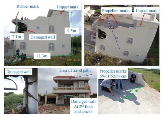
Figure 1.12-9 Initial aircraft impact, propeller, and rubber marks on building
