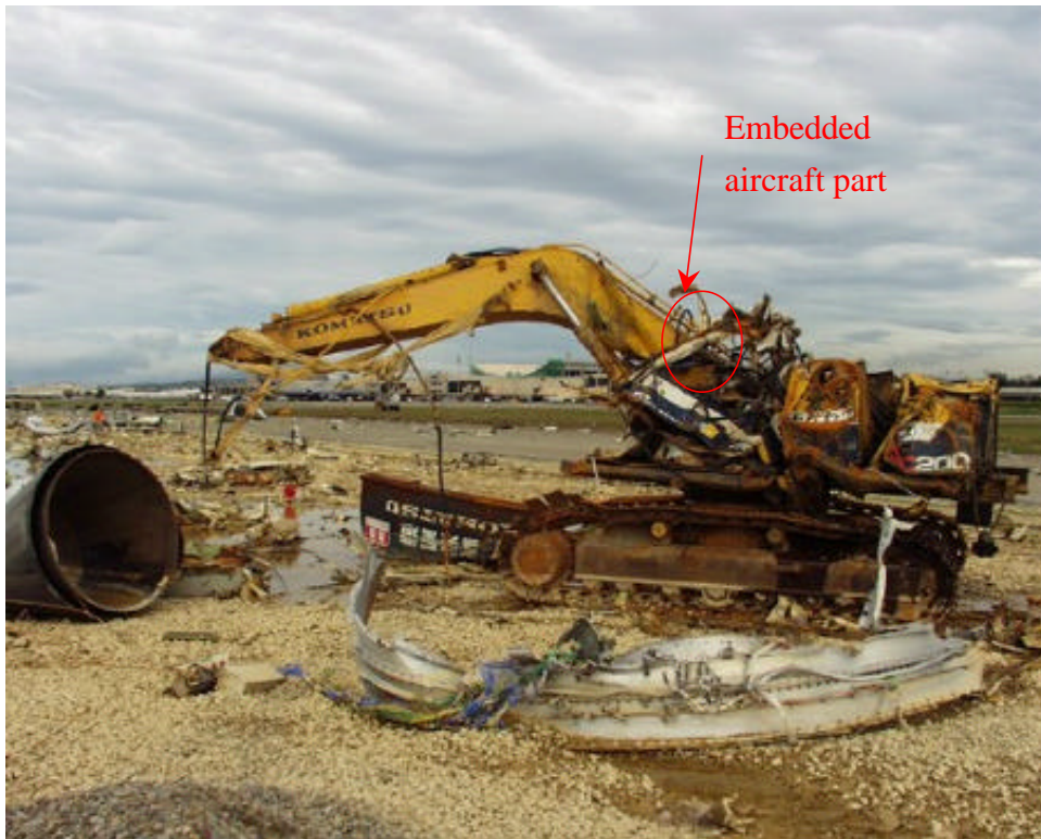
Fig. 1.4-2 Excavator ( in No.11 pit )
