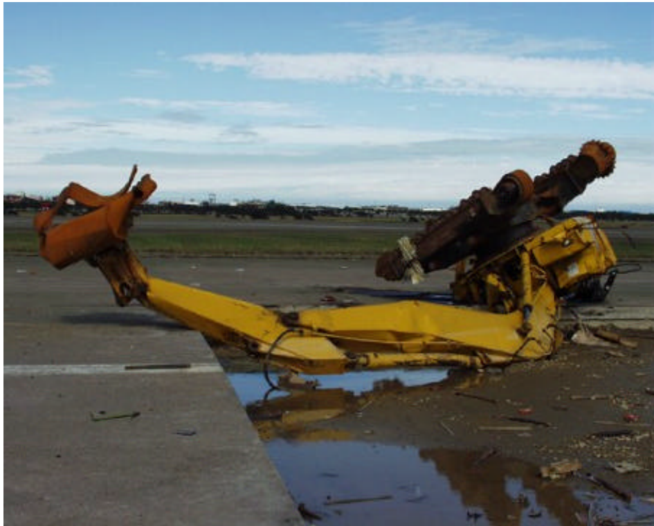
Fig. 1.4-1 Excavator ( in No.5 pit )
