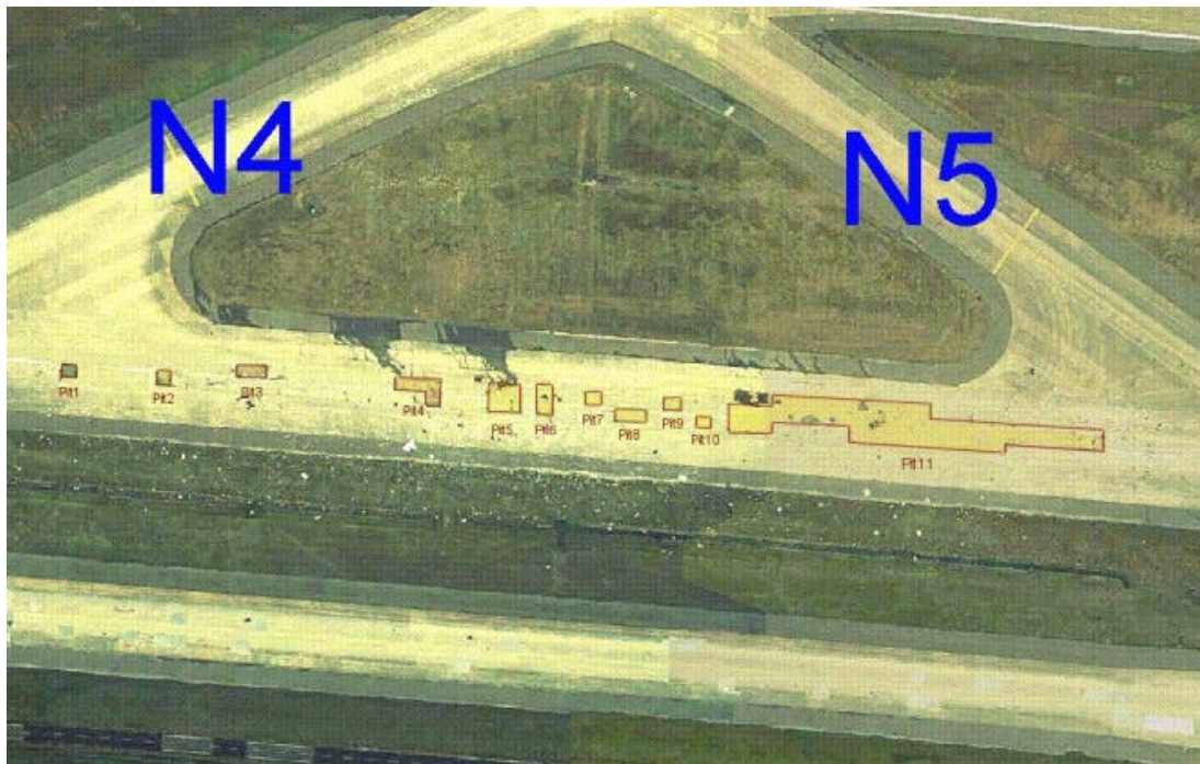
Fig.1.12.1-1 Removed Concrete Sections formed 11 different pits.
