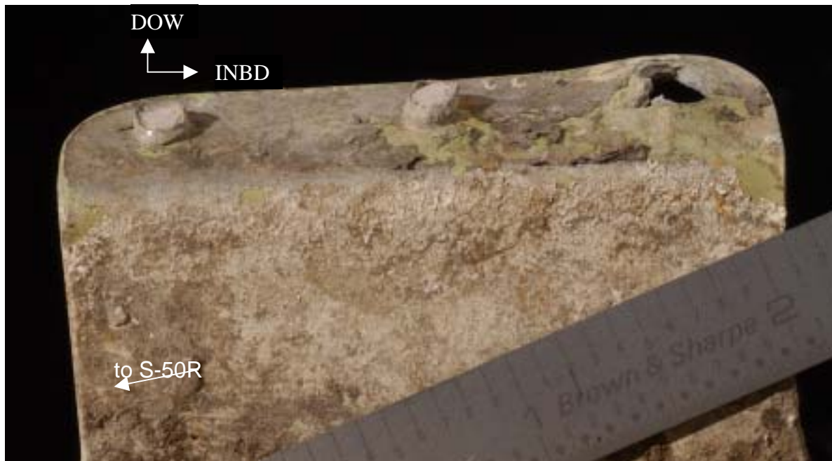
Figure 1.16-112 Shear tie between S-51R and S-50R of the STA 2100 frame segment showing downward deformation in skin flange and pull through of the fastener hole at the inboard most fastener hole.
