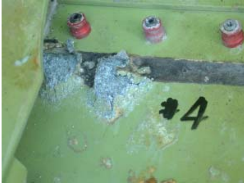
Figure 1.16-137 Higher magnification of #4 corrosion pit, before cleaning (1.27X)
