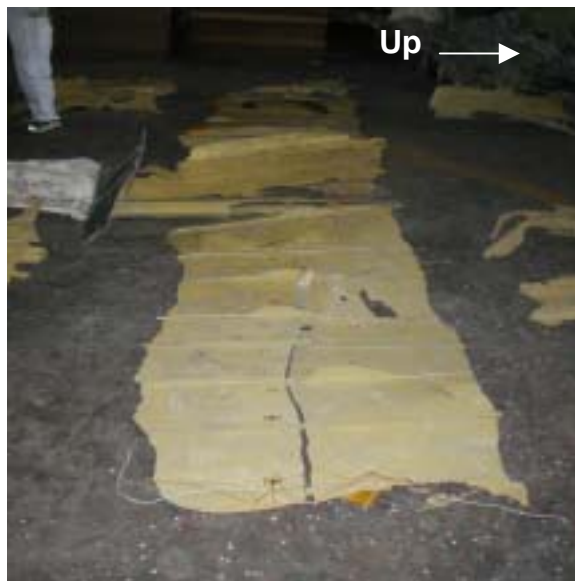
Figure 1.12-19 Aft side of Midspar viewed from right side
