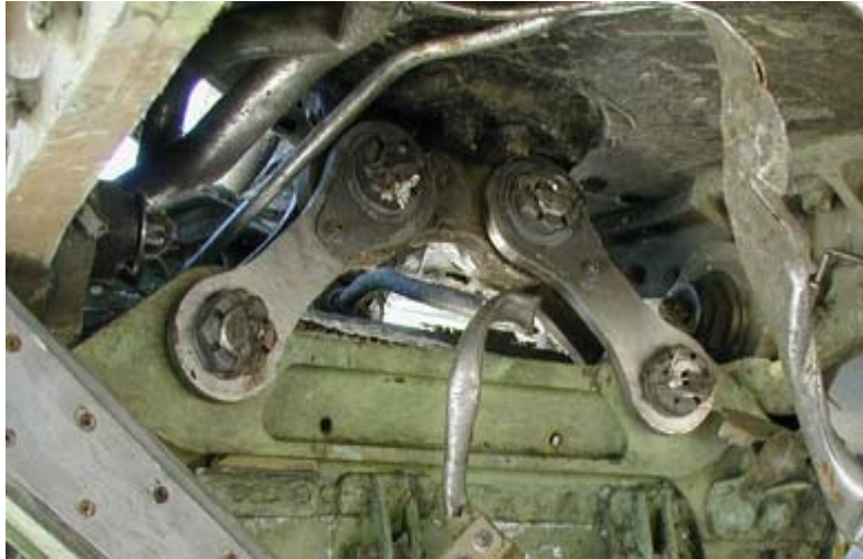
Figure 1.12-48 View of dual side links installed by strut modification
