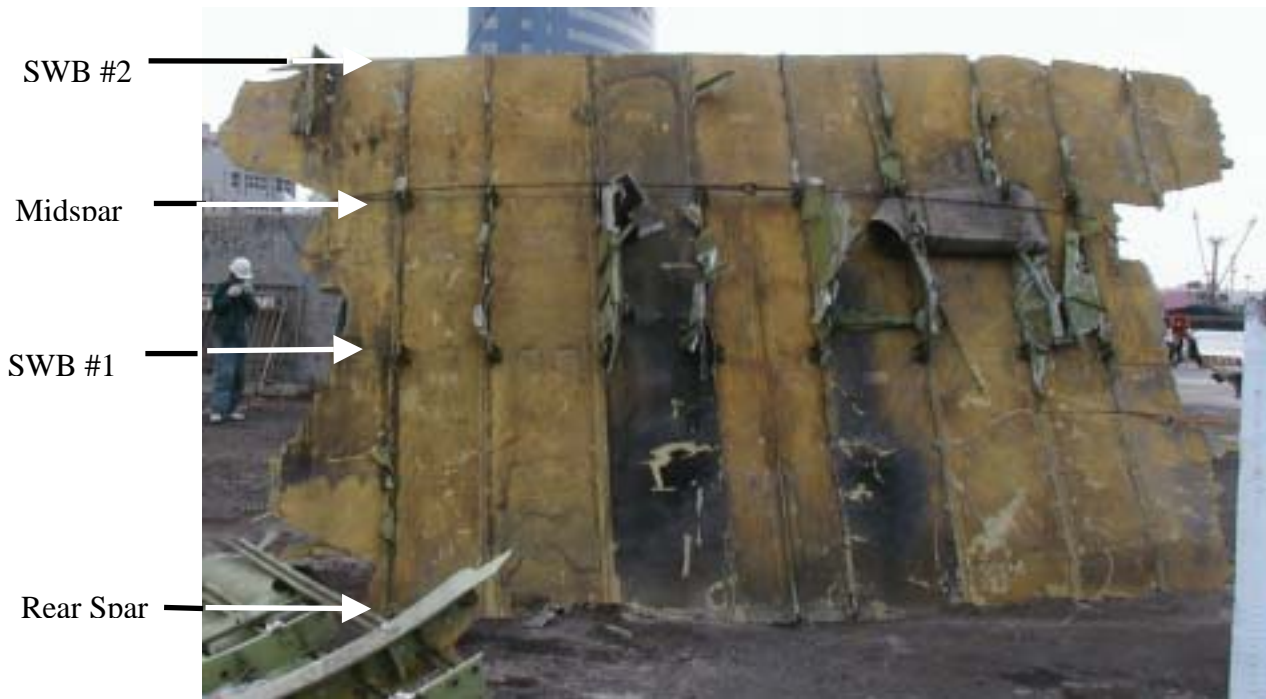
Figure 1.12-25 (a) Interior surface of Upper Panel Item #642-upper photo, (b) Exterior surface of Upper Panel Item #642-lower photo
