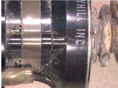
Figure 28: Detail view of switch #2, cracks in the body.
