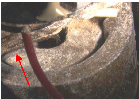
Figure 19: RIGHT, OUTFLOW VALVES Indicator; armature is over witness mark.
