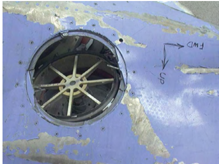
Figure 81: Upper Pressure Relief Valve, showing orientation, note that blowout doors are missing.
