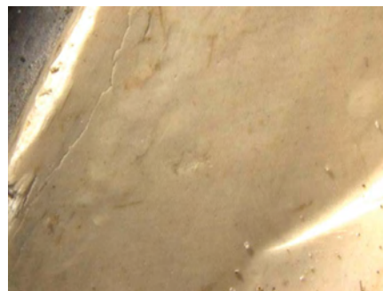
Figure 214: Lower Pressure Relief Valve; detail of valve gate, switch contact area.
