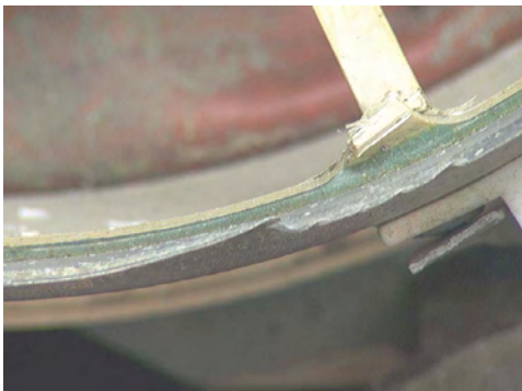
Figure 140: Close-up of knife-edge damage.
