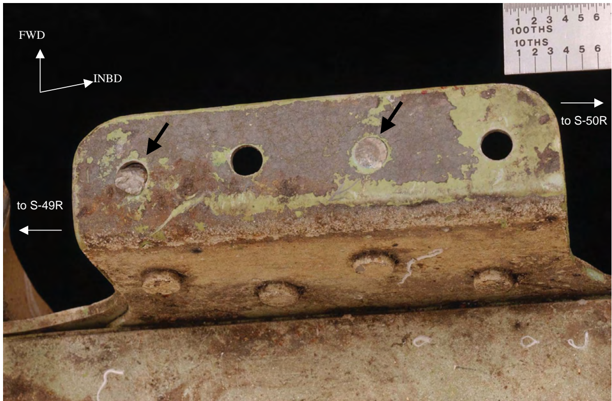
Figure 88. Skin flange rivet fractures at shear tie between S-49R and S-50R of the STA 2040 frame segment. Black arrows indicate the direction of loading.
