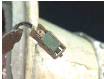
Figure 212: Switch (side view): actuator is missing from switch housing.
