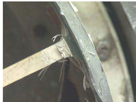
Figure 141: Close-up of knife-edge damage.
