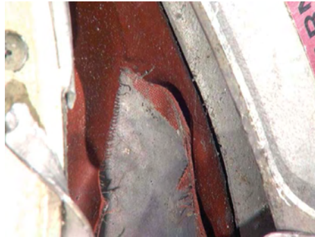
Figure 233: Outer diaphragm, close-up of tear origin.
