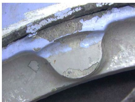
Figure 191: Upper stop pad; paint chipped.
