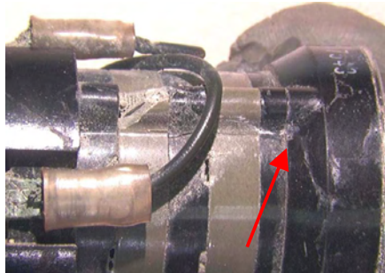
Figure 34: Bleed Air Switch #1.
