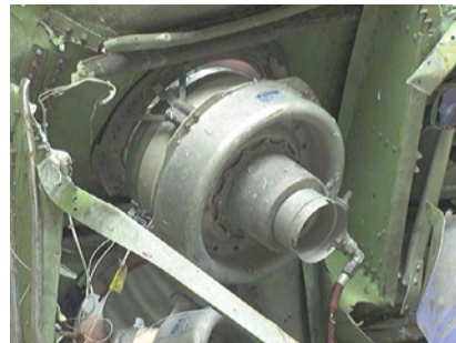
Figure 84: Upper Pressure Relief Valve still installed, as viewed from the inside.
