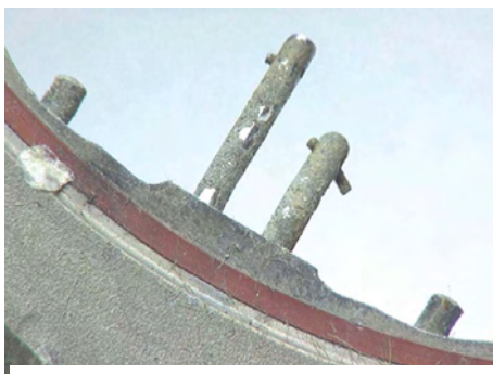
Figure 108: Close-up of aft stop & hinge pins (looking from inside out).
