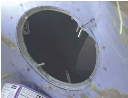
Figure 92: Upper Pressure Relief Valve, pins in approximately "door closed" position.
