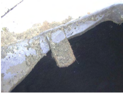
Figure 125: Overview of aft/upper stop pin as viewed from outside.
