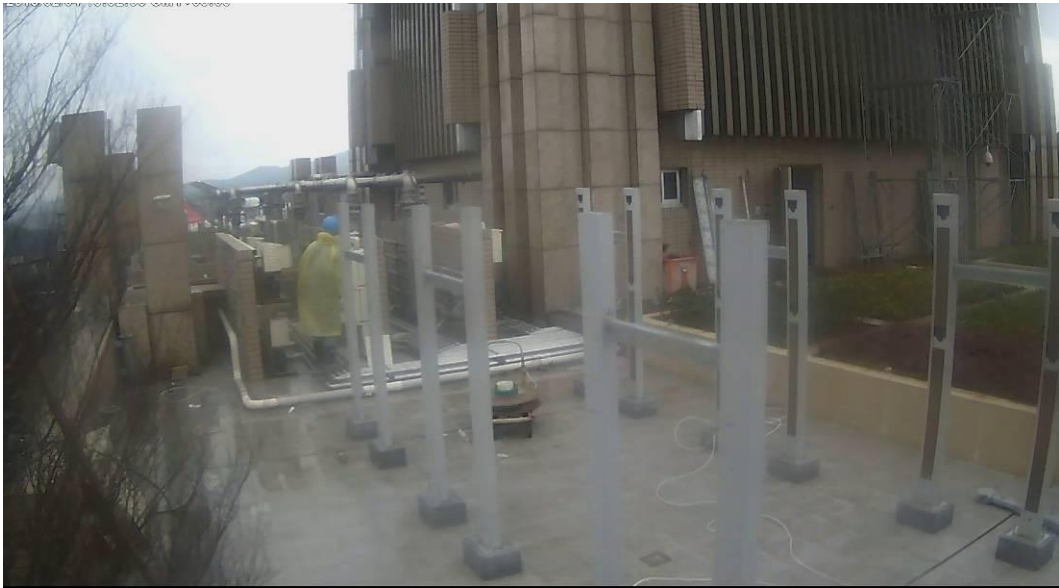
Figure 1.12-14 Surveillance video snapshot of channel 32 in building A
