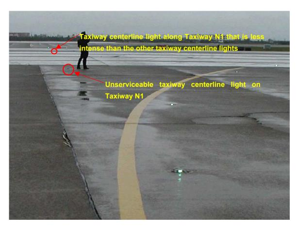
Figure 1.10-10 Status of Taxiway N1 centerline lights close to the threshold of Runway 05R (picture taken on November 4, 2000)
