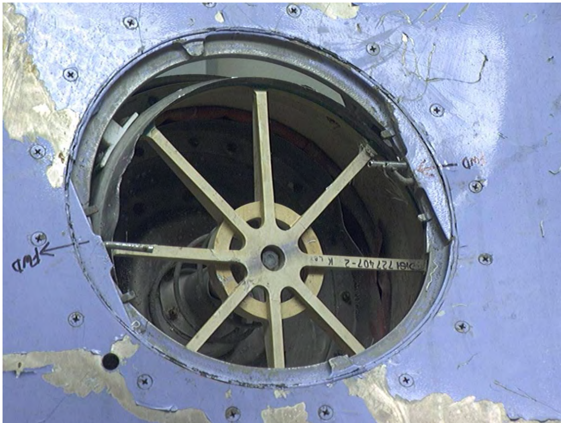
Figure 2.7-5 Upper pressure relief valve
