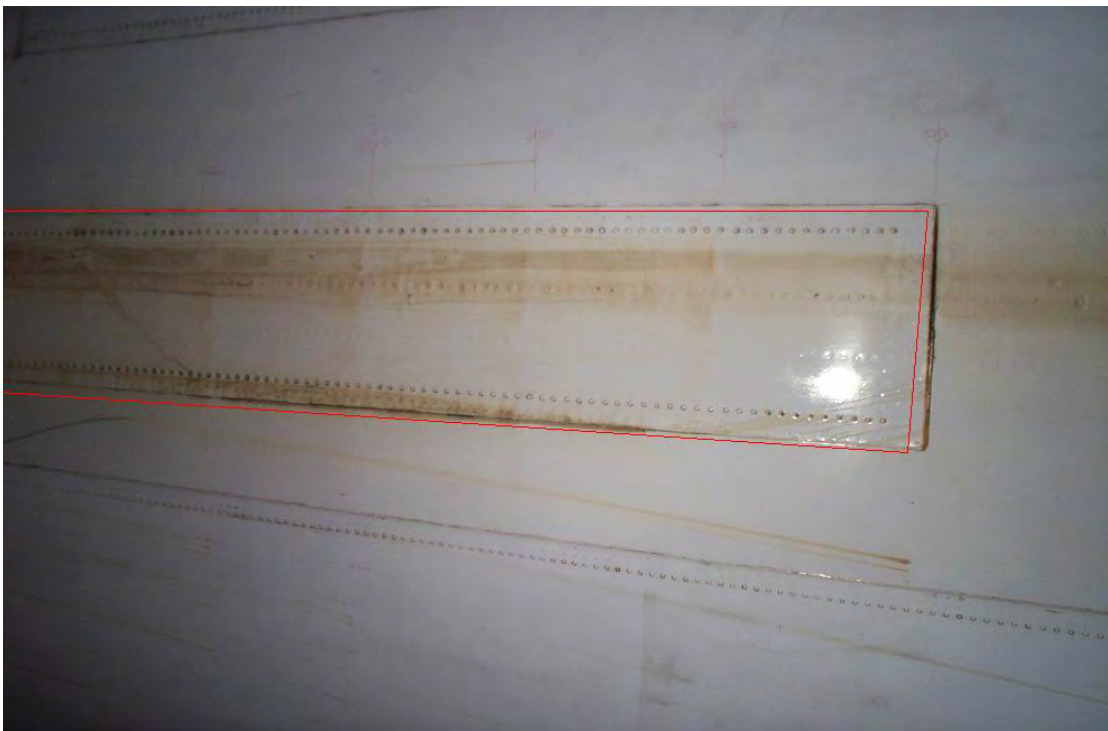
Figure 1.6-9 Fwd of No. 16 doubler (Picture taken on Nov 26,2001)
