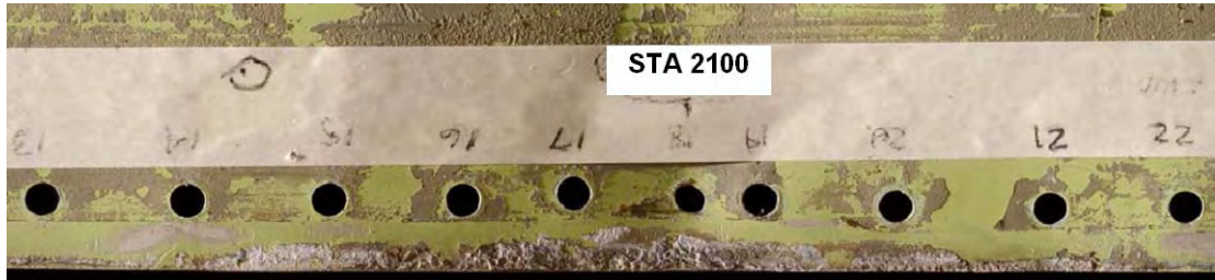
Figure 1.16-6 Light colored deposit on the faying surface of the repair
