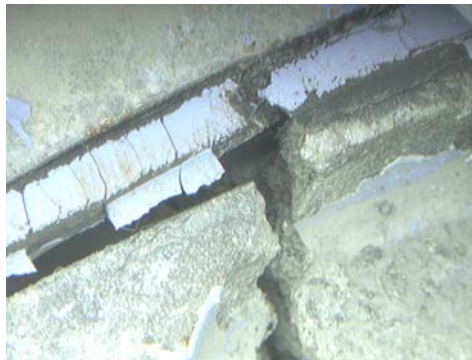
Figure 201: Detail of lower stop pad.
