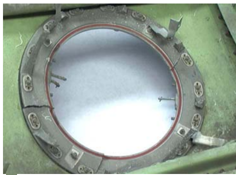
Figure 91: Interior view of opening with valve removed (looking inside to outside).
