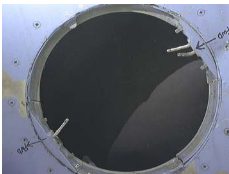
Figure 94: Upper Pressure Relief Valve, pins in approximately "door fully open" position.
