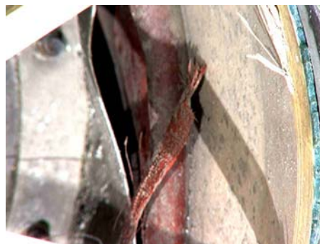
Figure 145: Diaphragm, 75 % of outer circumference is torn/split.
