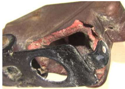
Figure 62: Bottom view of switch guard damage.
