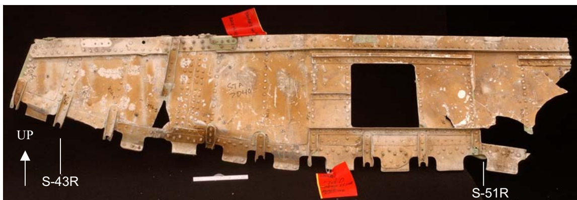
Figure 85. As received condition of the STA 2040 frame segment submitted for examination. The forward surface is shown in this view.
