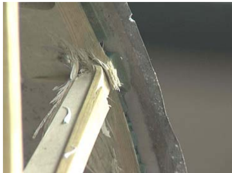
Figure 143: Close-up of web, representative of web fractures at gate ID.
