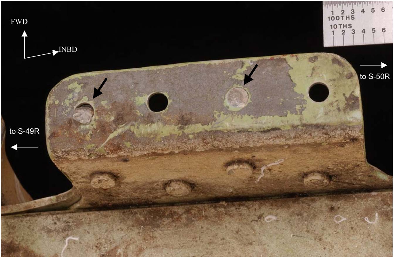
Figure 88. Skin flange rivet fractures at shear tie between S-49R and S-50R of the STA 2040 frame segment. Black arrows indicate the direction of loading.
