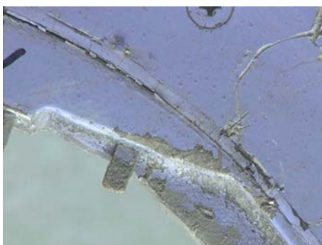
Figure 135: Overview of aft/lower stop pin, exterior view.
