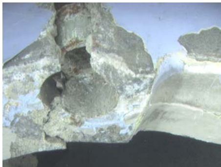
Figure 186: Forward/upper hinge pin bushing hole. • Housing is cracked and contains partial bushing.
