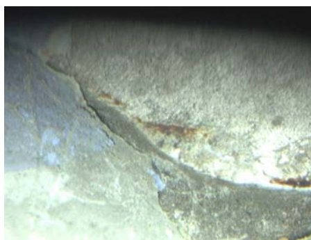
Figure 203: Close-up of figures #200 and #202, slight dent on pad, paint chipped.
