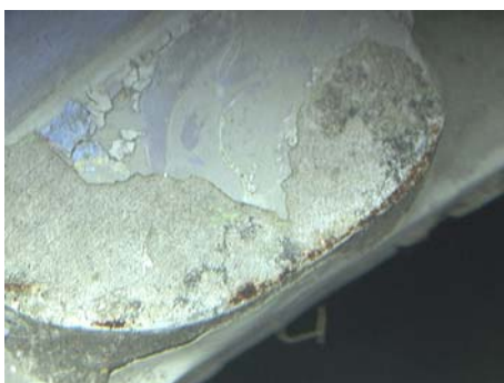
Figure 202: Close-up of figure #200, paint chipped.
