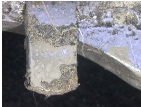
Figure 137: Aft/lower stop pin, close-up of figure #136. • Paint is chipped.
