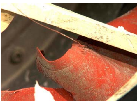
Figure 227: Outer diaphragm HS P/N 727403-1, torn location.
