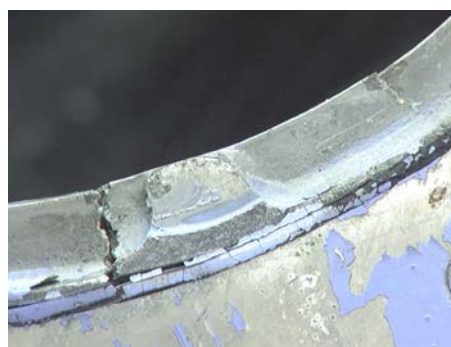
Figure 190: Exterior opening, close-up, upper door stop pad.
