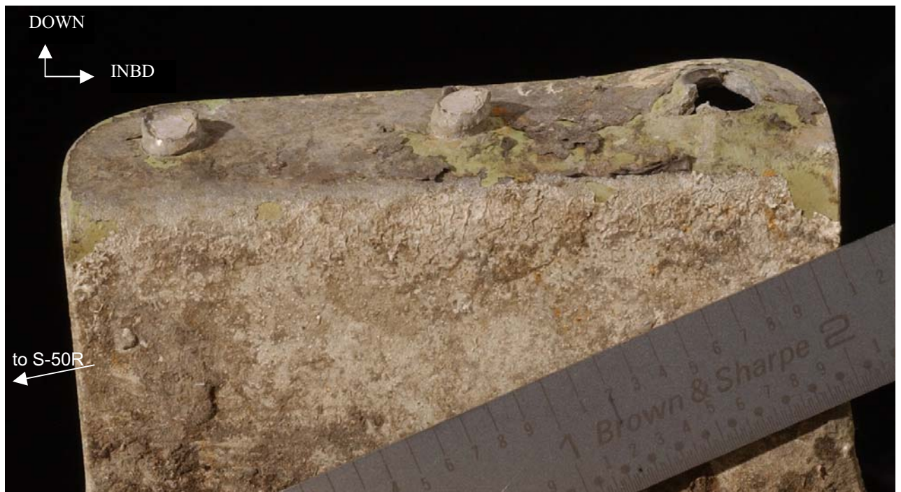
Figure 78. Shear tie between S-51R and S-50R of the STA 2100 frame segment showing downward deformation in skin flange and pull through of the fastener hole at the inboard most fastener hole.
