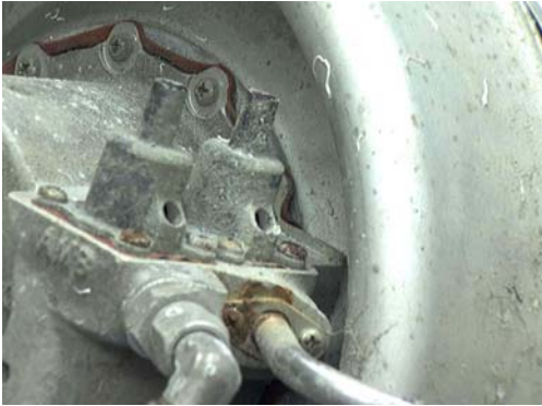
Figure 157: Exterior view of sensors, showing some apparent corrosion on the integral ambient sense tube.
