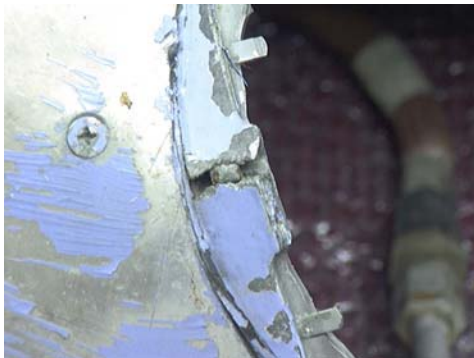
Figure 184: Exterior opening, close-up of fracture of valve housing at forward/upper hinge pin.
