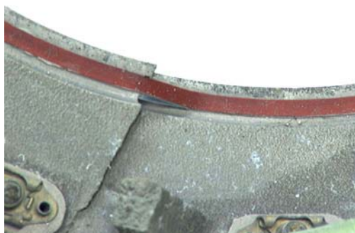
Figure 99: Another cut on the seal.
