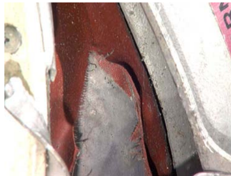
Figure 233 : Outer diaphragm, close-up of tear origin.
