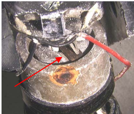
Figure 17: LEFT, OUTFLOW VALVES Position Indicator witness mark
