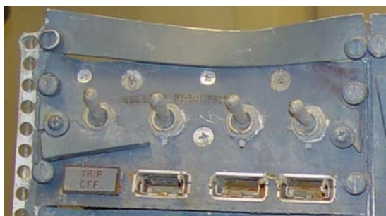
Figure 52: Galley Power control panel M179 • Light plate is missing. • All switch toggles are in up position. • TRIP OFF indicator lights, numbers 2, 3 & 4 legend plates, bulbs and retaining assemblies are missing.
