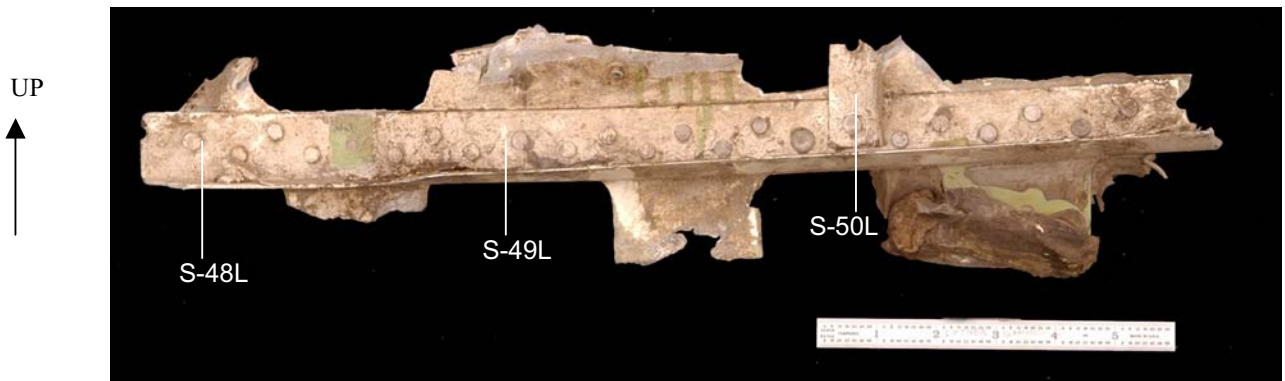
Figure 71. As received condition of the STA 2160 frame segment submitted for examination. The aft surface is shown in this view.
