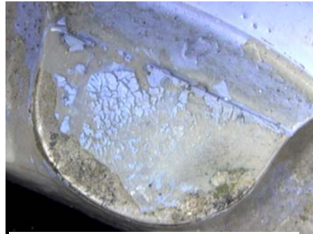
Figure 116 : Upper stop, pad, close-up of figure #115.
