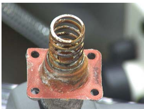
Figure 171: Integral ambient sensor spring & diaphragm. • Heavy hardened corrosion on spring and diaphragm in localized areas. • Corrosion on spring seat almost all the way around.
