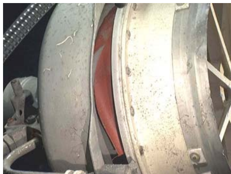
Figure 148: Diaphragm, circumferential tear.
