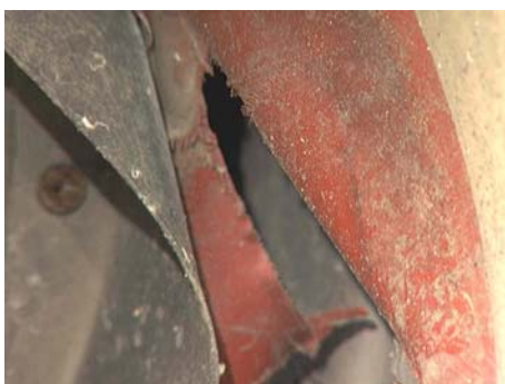
Figure 228: Outer diaphragm, approximately 60% of circumference is torn.
