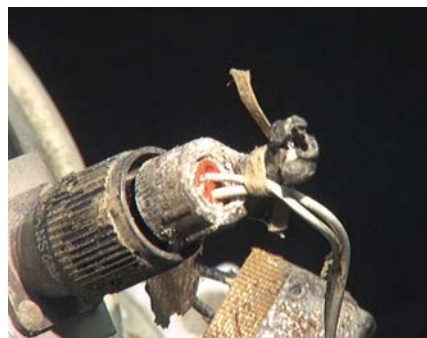
Figure 210: Electrical switch connector interface appears to be intact.
