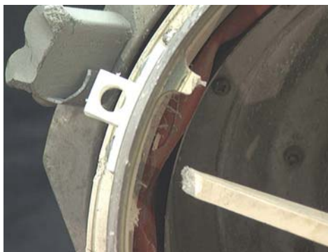
Figure 217: Broken web detail.
