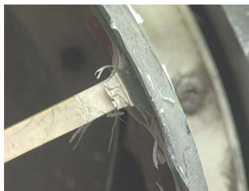
Figure 141: Close-up of knife-edge damage.
