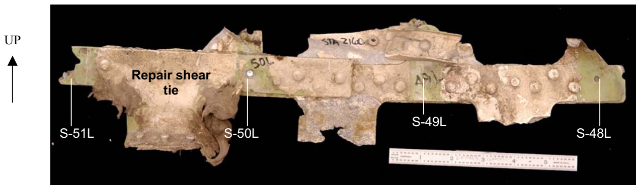
Figure 72. As received condition of the STA 2160 frame segment submitted for examination. The forward surface is shown in this view.
