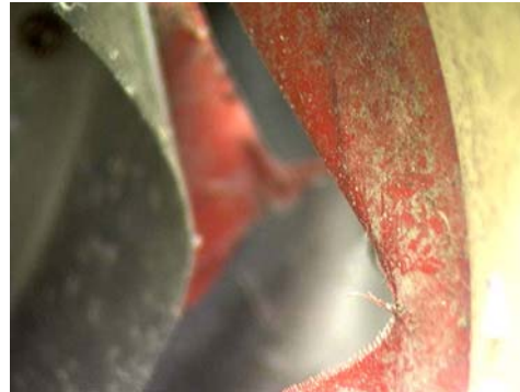
Figure 231 : Outer diaphragm damage.
