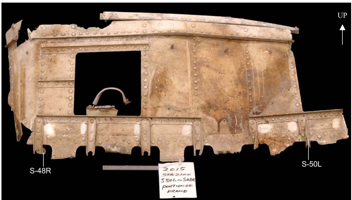
Figure 76. As received condition of the STA 2100 frame segment submitted for examination. The forward surface is shown in this view.
