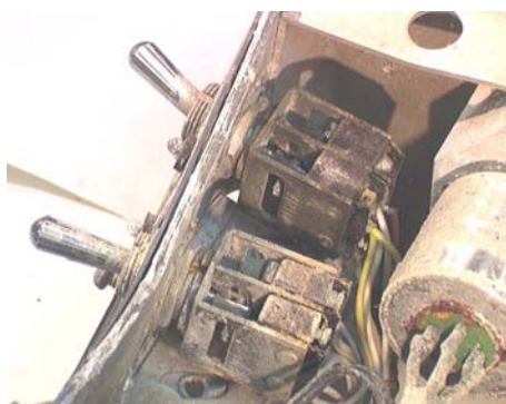
Figure 22: Outflow Valves, MANUAL CONTROL, OPEN & CLOSE toggle switches as viewed from underneath.
