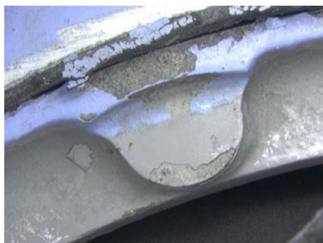
Figure 191: Upper stop pad; paint chipped.
