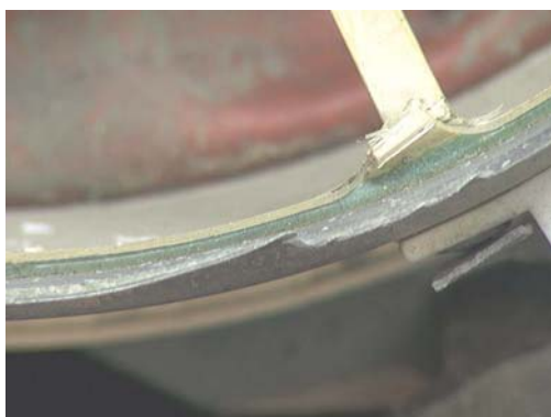
Figure 140: Close-up of knife-edge damage.
