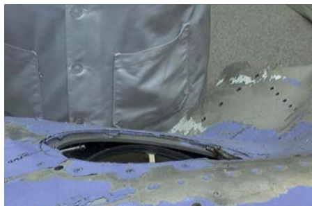
Figure 77: Upper pressure relief valve, (center of picture) distorted exterior skin.
