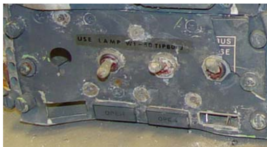
Figure 67: DC BUS ISOLATION panel, module M557
