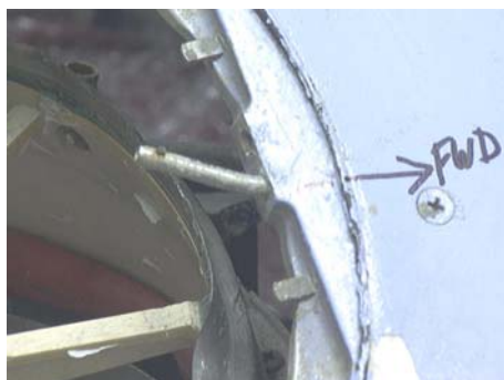
Figure 113: Forward/upper hinge pin, upper door (forward/lower hinge pin is missing).
