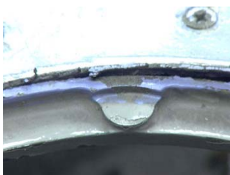
Figure 189: Exterior opening, close-up, upper door stop pad.
