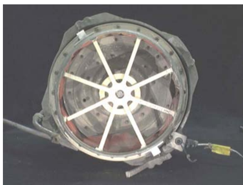
Figure 138: Overview of valve face. • Knife-edge has some rolled over areas and some bent edges. • In general, reasonably round. • 2 gate spacers, HS P/N 727407-30 are missing, remaining 2 spacers on top and bottom as shown.
