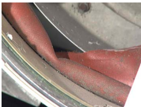
Figure 146: Diaphragm, showing typical tear.
