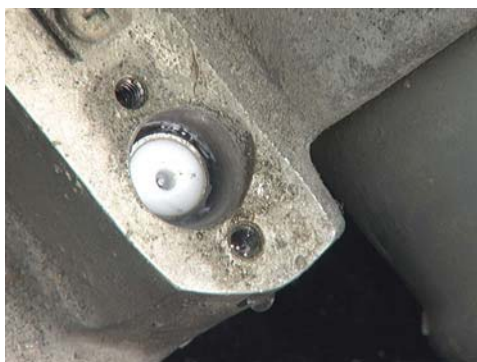
Figure 169: Shows water in plug area.
