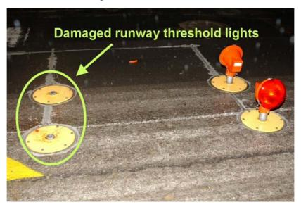
Figure 1.4-1 Damaged runway threshold lights
