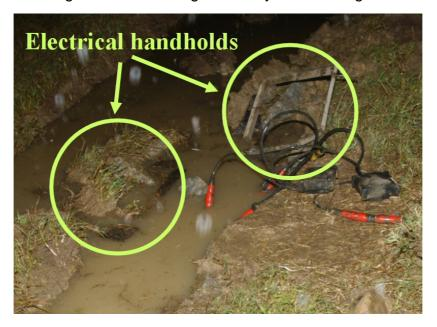
Figure 1.4-2 Damaged electrical handholds
