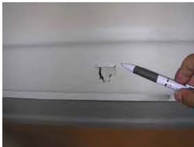
Figure 1.12-3 A puncture on a ceiling panel.
