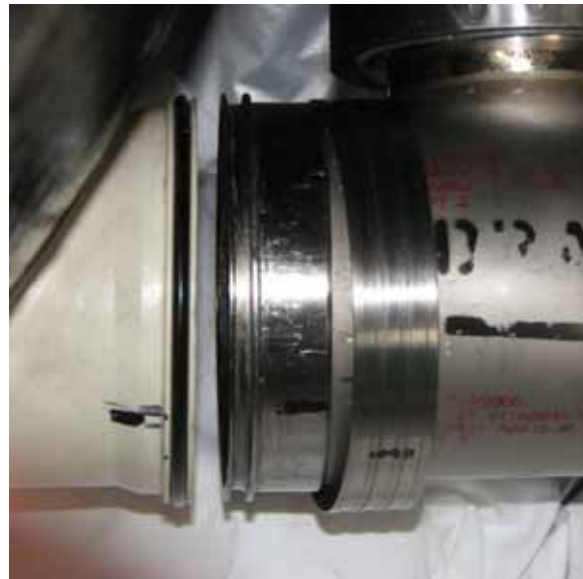
Figure 1.18-2 Photo of Waste Tank Outlet and Coupling Short Tube
