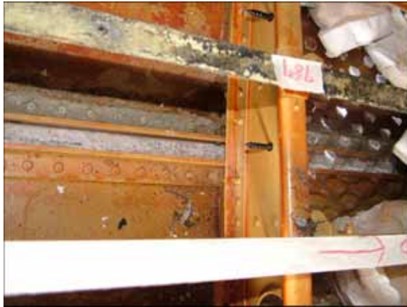
Figure 1.12-2 (C) Corrosion aft of Sta. 787
