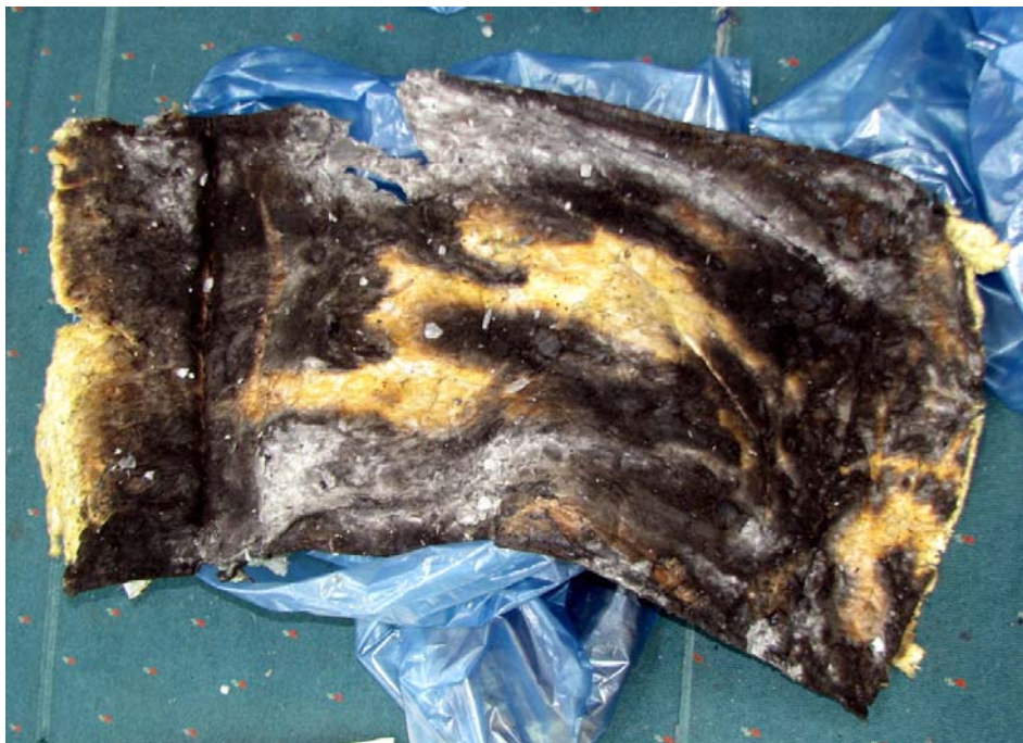
Fig. 1.12-10 Charcoaled with Grayish Deposit on Insulation Core Layer
