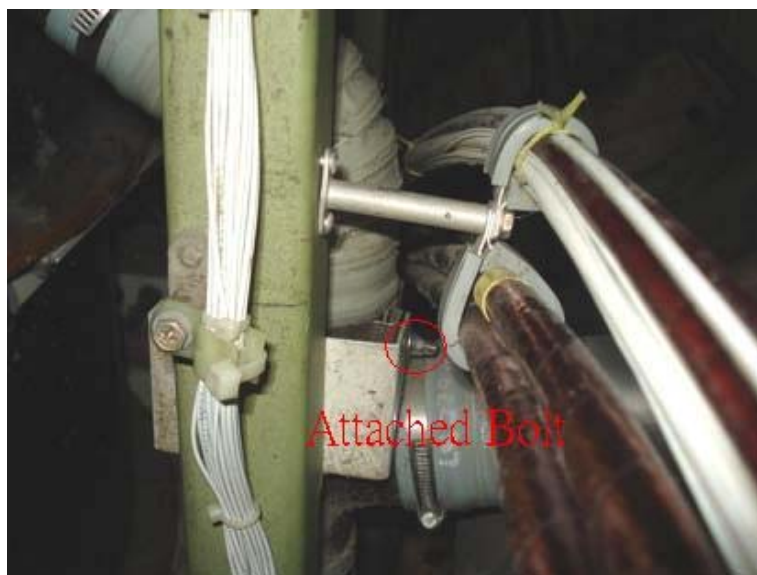
Fig. 1.14-1 Attached Bolt of Waste Tank Tube Fixture
