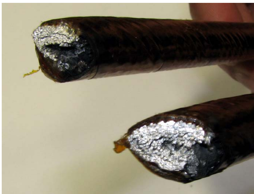
Fig. 1.12-21 Cut through View of the Damaged Spot of the Cable
