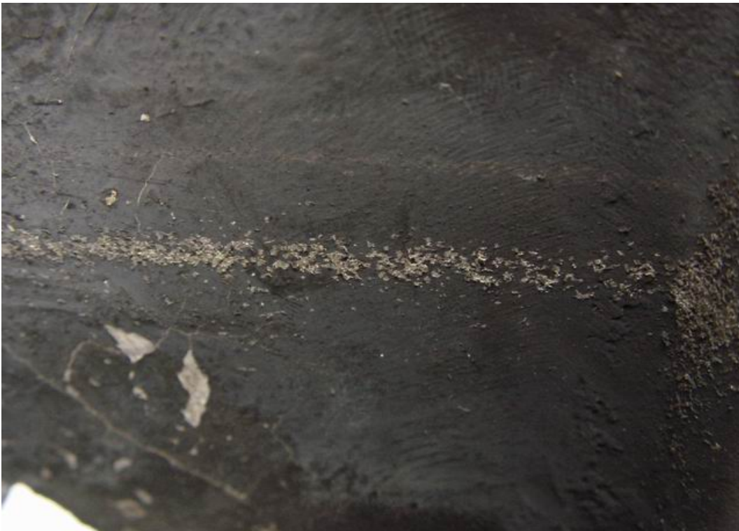
Figure 2.3-6 The melted metal of the impeller was flung outward by centrifugal force and adhered to the inner wall of the rear inlet case
