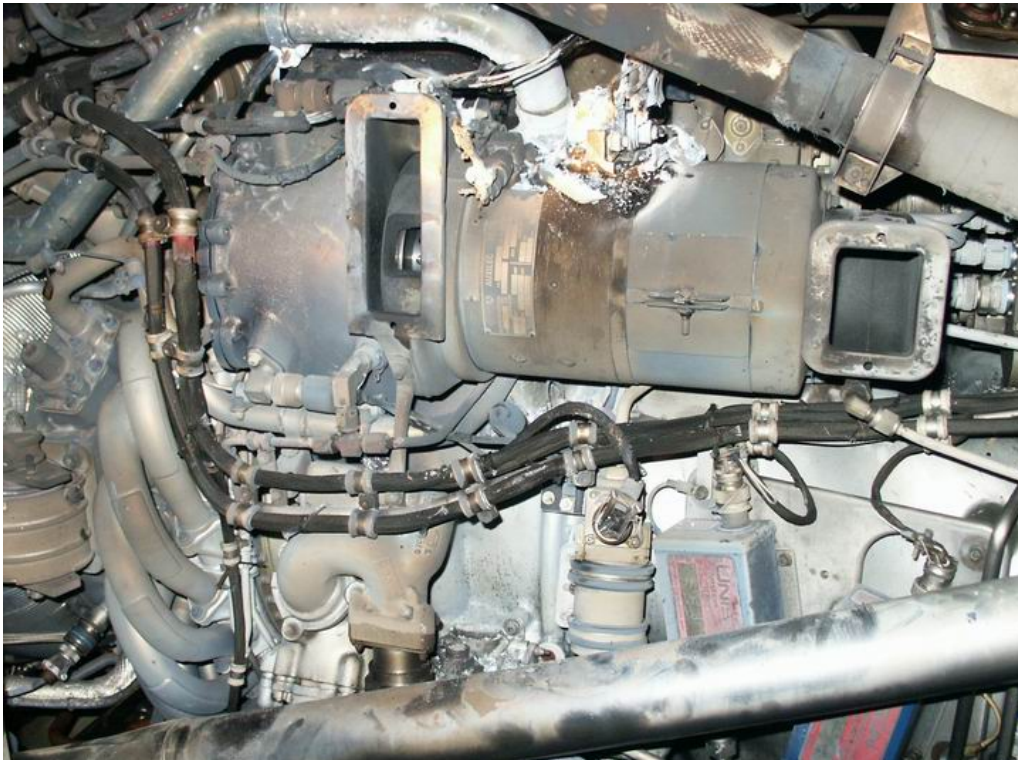
Figure 1.2-1 DC starter generator wire protection cover
