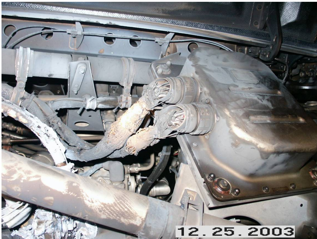
Figure 1.7-1 Part of the fire damaged wiring
