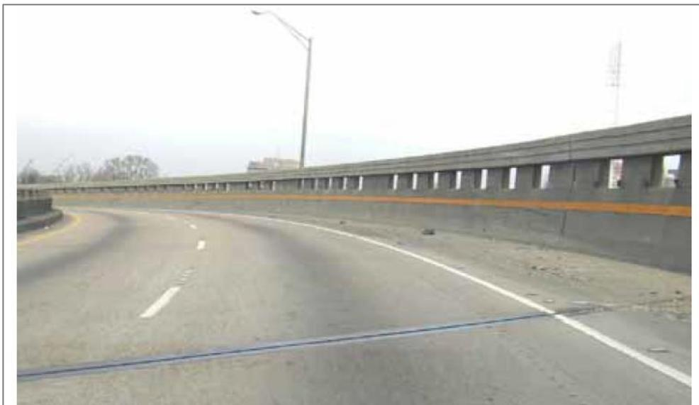
Figure 7-6. Texas Type TT Railing
